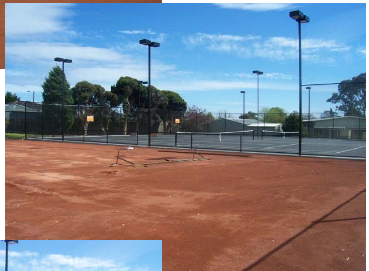
View of Courts 5/6 & Court 4
