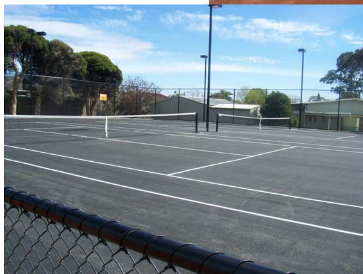
Courts 5 & 6 – new surface, new lighting
