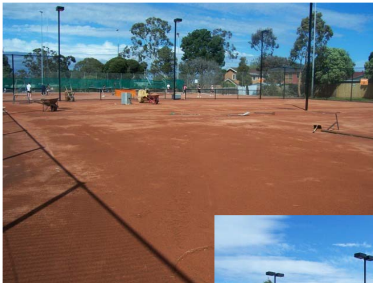
Courts 3 & 4 – under repairs, new lighting
